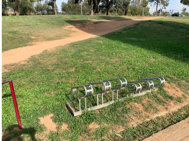
Figure 1. Installation of bicycle and electric scooters parking
